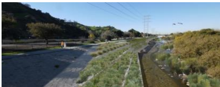
Reach 5 Channel Terracing
