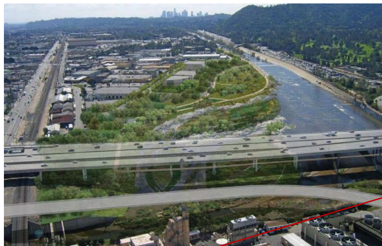
Reach 3 Verdugo Wash
