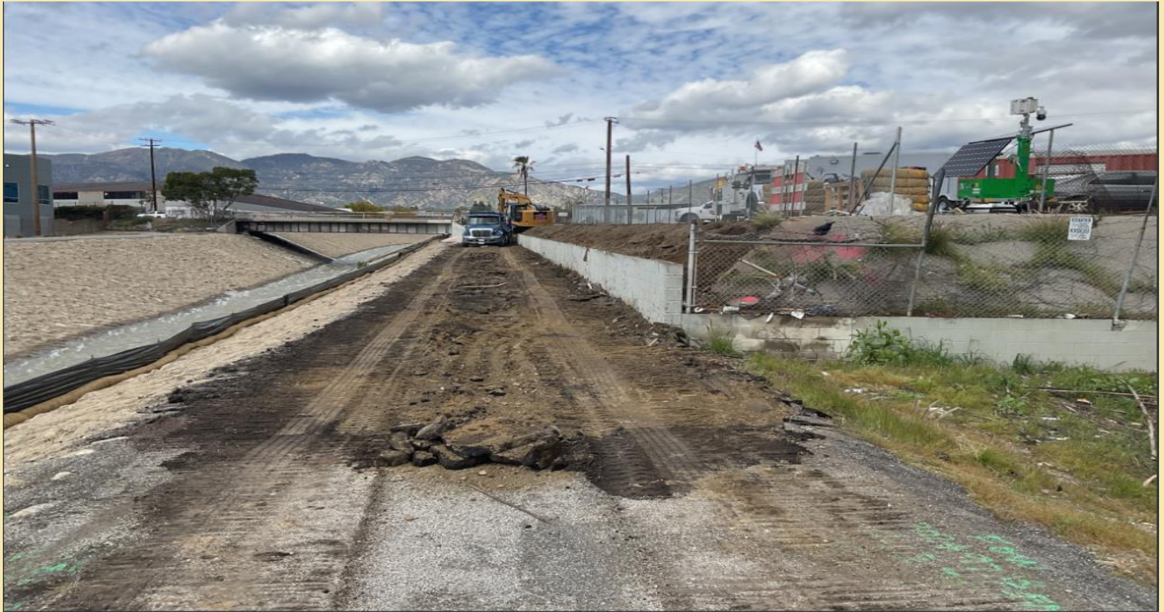
Excavation for retaining walls D1 and D2 south of Fifth Street
