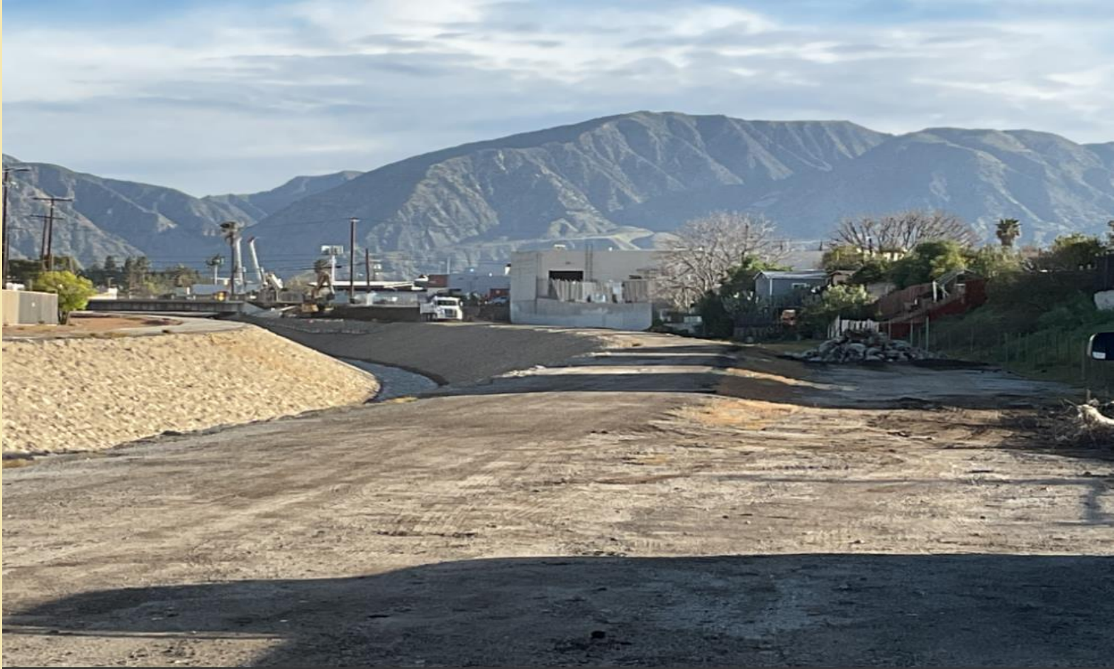
View of future bikeway and bioswales from Bradley Avenue
