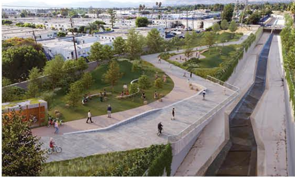
ALISO - Wilbur Debris Basin
