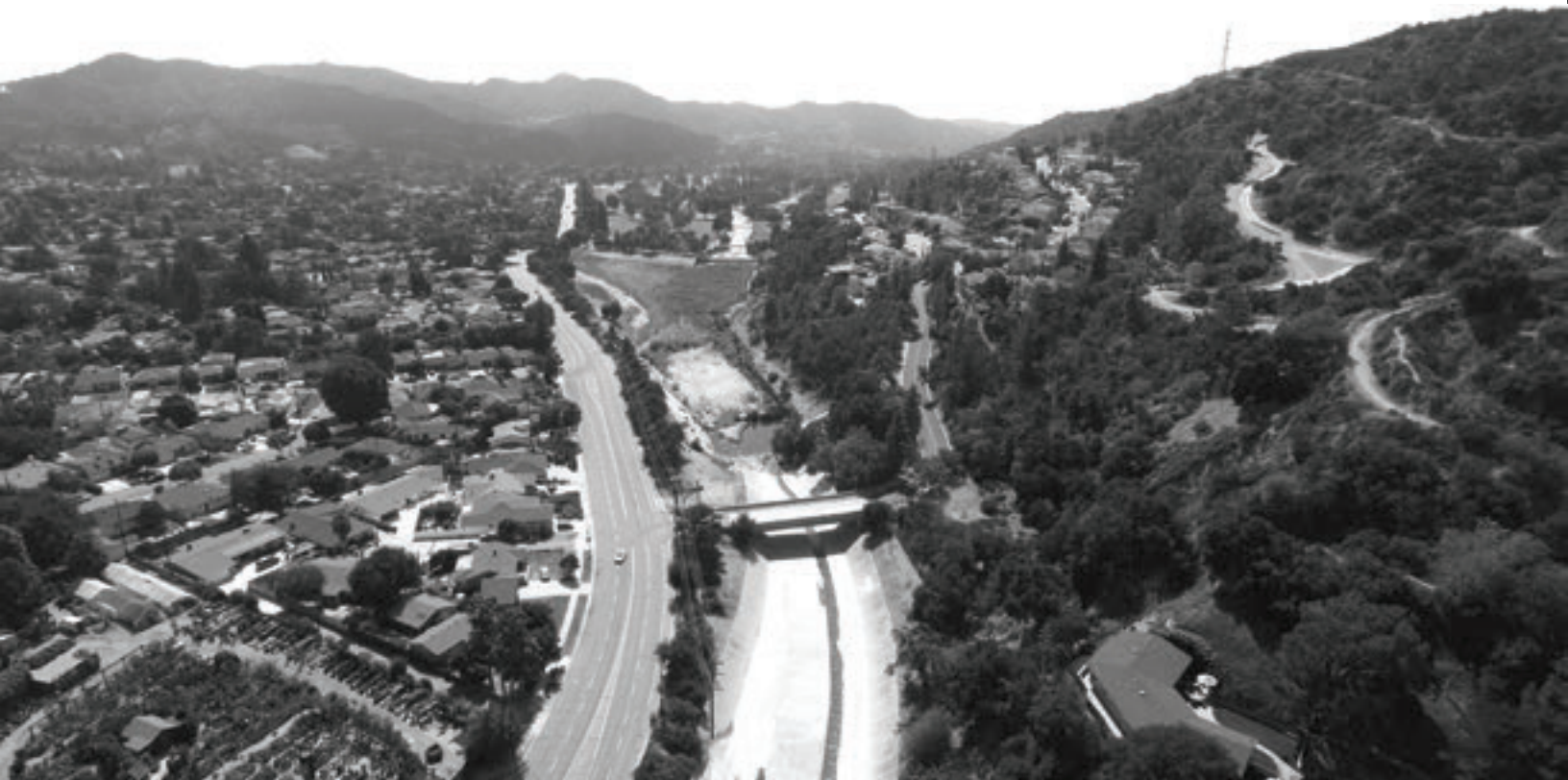
View looking south at Verdugo Wash and Invale Drive
