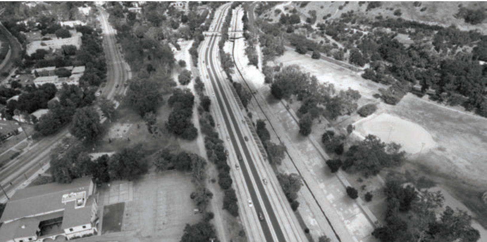
View looking north at the Arroyo Seco near the Montecito Recreation Center
