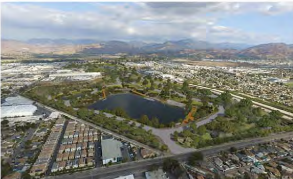
TUJUNGA - Hansen Dam Spreading Grounds
