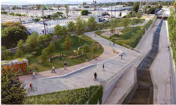
ALISO - Wilbur Debris Basin
