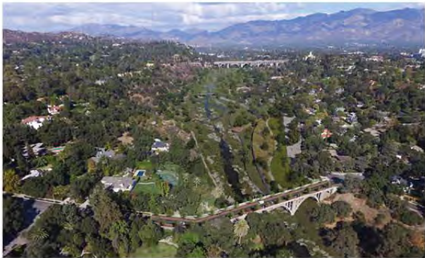
ARROYO SECO - Lower Arroyo Park
